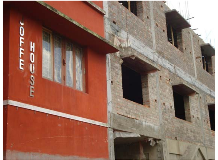
Extension part of Joffe House(Under construction)
